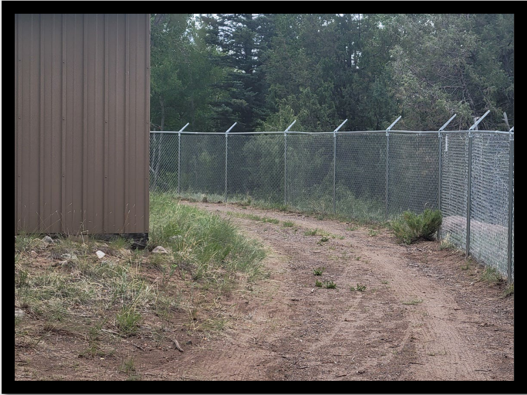
New Fence at S. Crestone Tank
