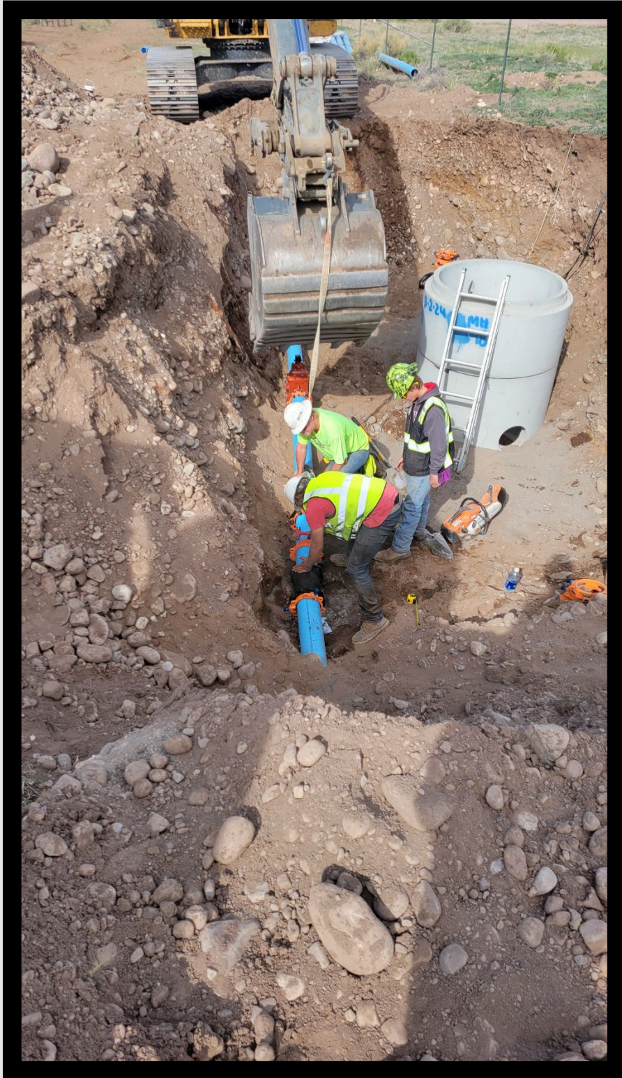
New Meter Vault Being Installed
