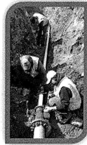
3" Water Main Repair
