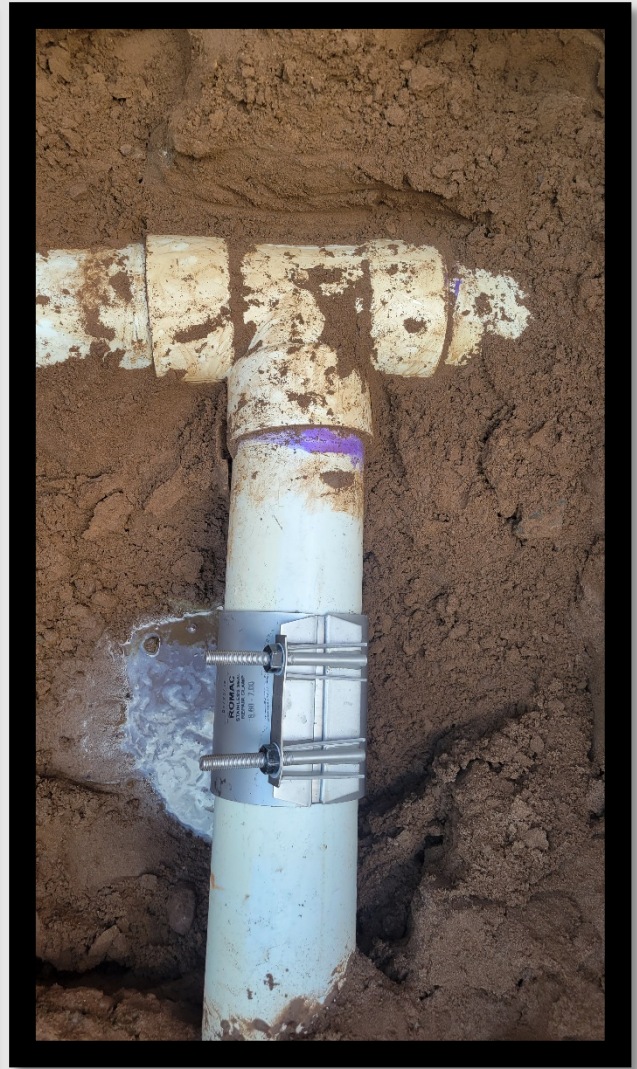
Repair of water main break on Camino Baca Grande.
