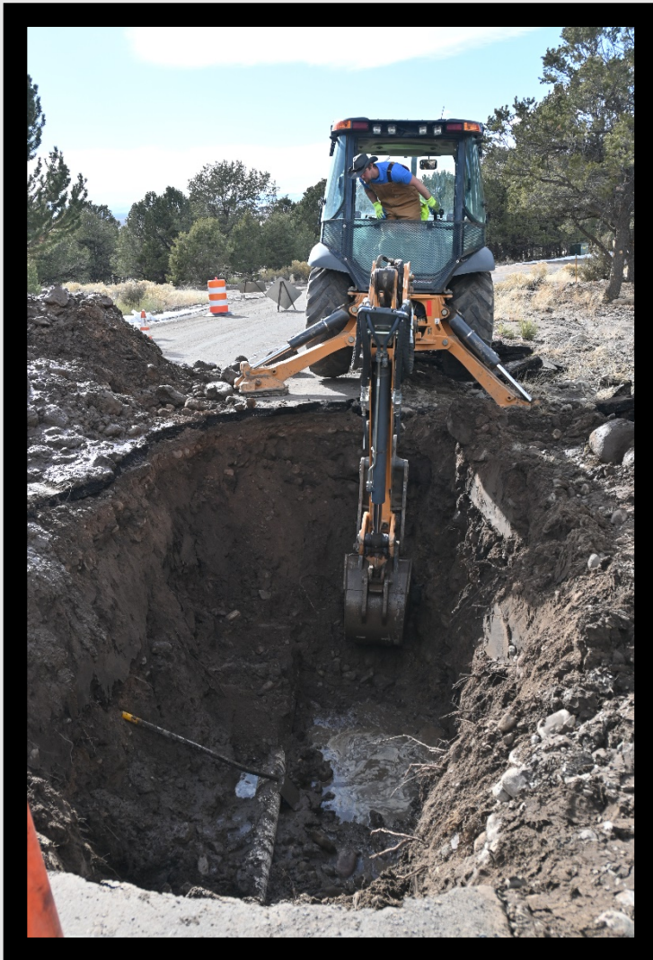
Operations Staff excavating water main break on Moonlight Overlook
