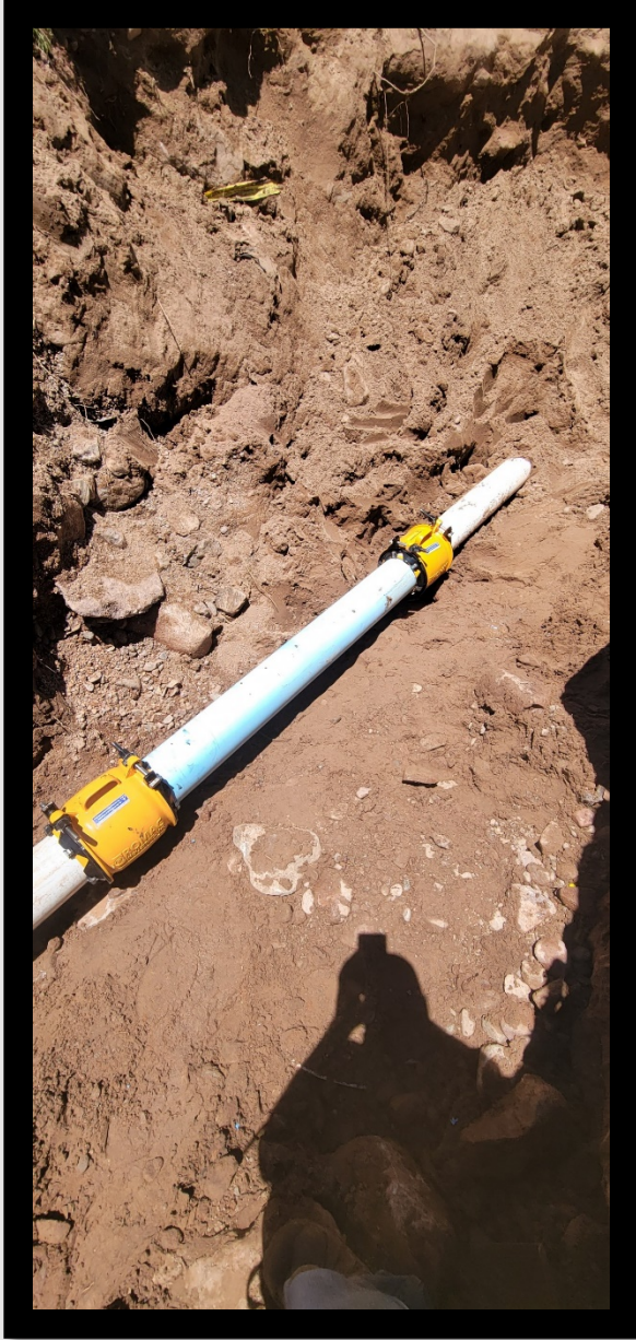
Picture of the water main break and repair on July 4 th , 2022.
