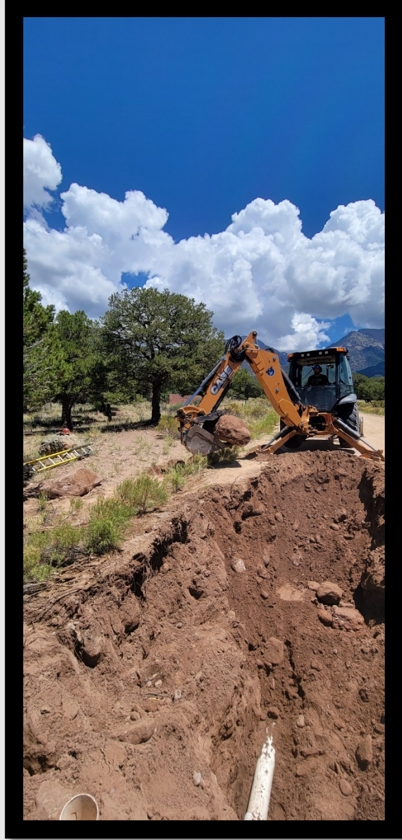
Picture of the water main break and repair on July 4 th , 2022.
